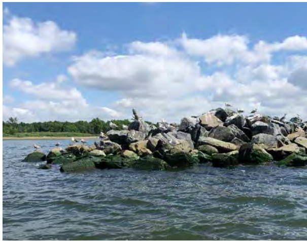
LIVING BREAKWATERS Just across Raritan Bay in Tottenville, Staten Island (NY), living breakwaters are being constructed to reduce long-term beach erosion, knock down storm waves, and provide structured habitat for a variety of aquatic species. (Image Credit: SCAPE)
