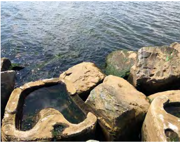
LIVING BREAKWATERS Just across Raritan Bay in Tottenville, Staten Island (NY), living breakwaters are being constructed to reduce long-term beach erosion, knock down storm waves, and provide structured habitat for a variety of aquatic species. (Image Credit: SCAPE)
