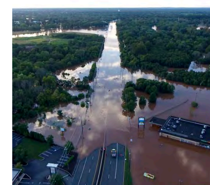
Raritan, NJ - Hurricane Ida - Remnants of Hurricane Ida created widespread flooding along areas of Route 206 and surrounding roads in Somerville and Raritan. Source: Iola Register.
