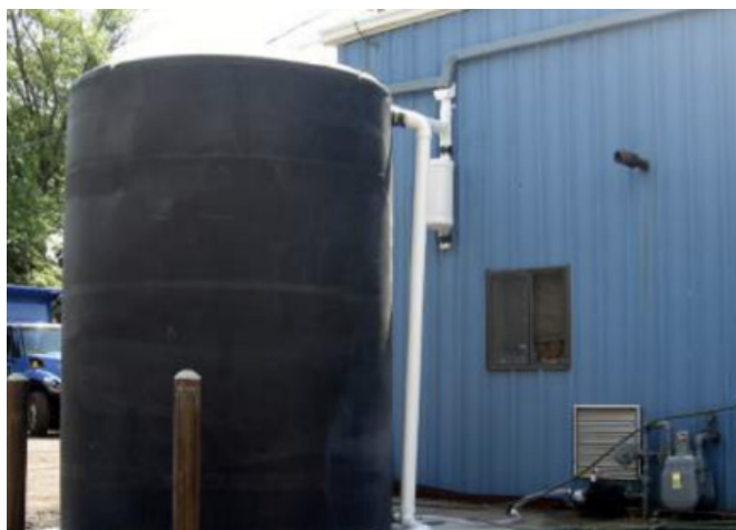
Fig.28. A cistern installed at a public works department in Clark, NJ. The rainwater is harvested from the rooftop of the building and used as part of a green car wash system.
